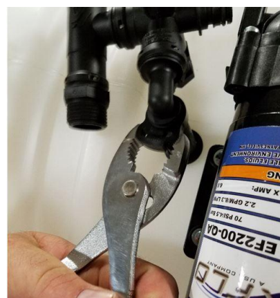
Figure 6 Use Pliers to tighten F-size Clamp as shown to secure Return Line.
